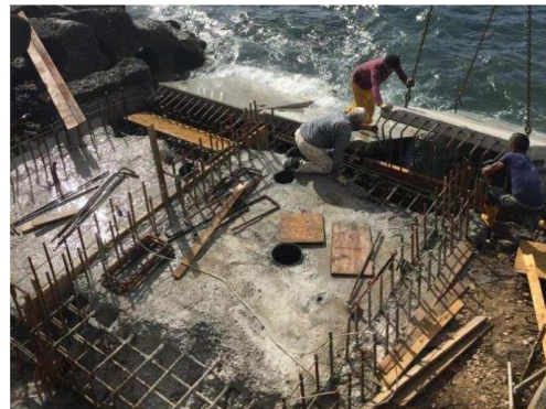
Fig. 9 - Positioning of the prefabricated ramps
