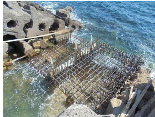
Fig. 8 - The bottom slab construction
