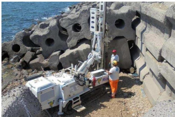
Fig. 7 - Construction of micropiles by micropiles drilling rig
