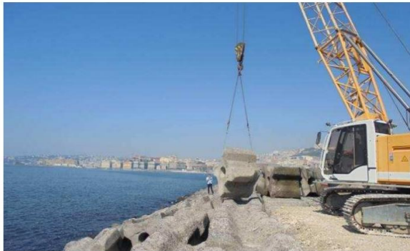
Fig. 6 - Antifers handling by mobile crane
