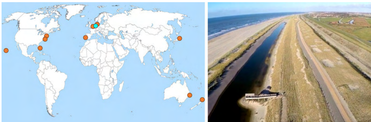
Left: a map of the hybrid dune cases in the inventory. Blue dot: the Hondsbossche Sea Dike, shown on the right
